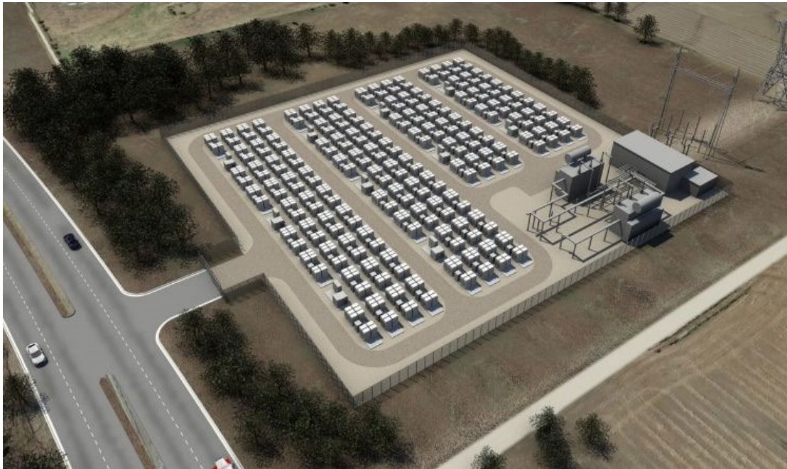
FIGURE 7-5 SOLARCITY'S TESLA BATTERY STORAGE FACILITY, HAWAII
