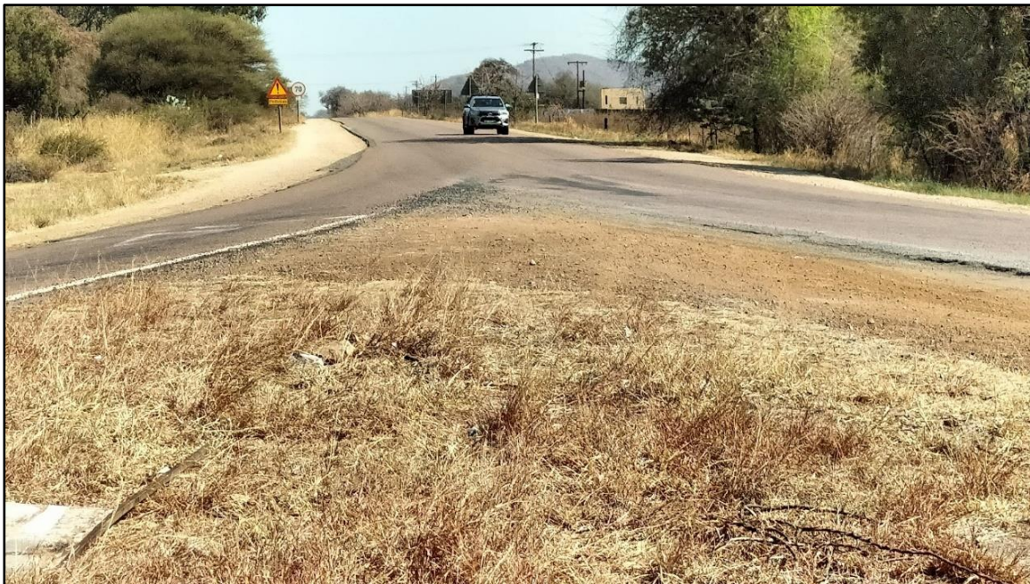
View along D114 on its approach to R565
