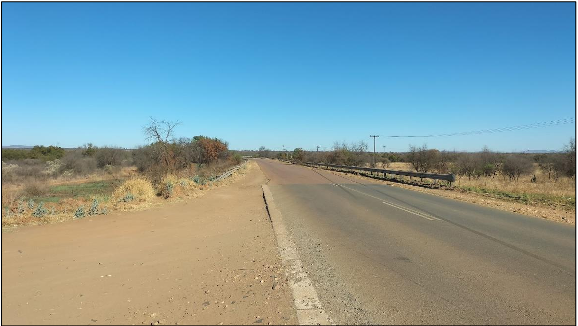
View to left of gravel site access road intersection with D114
