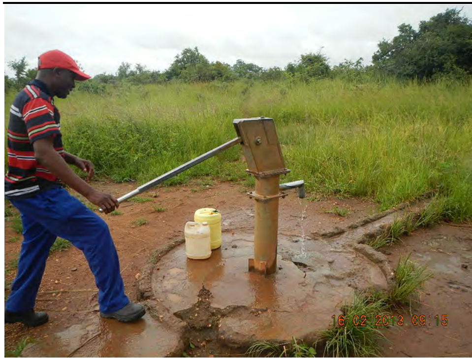
Figure 4.18 A Typical Hand Pump in the Project Area
