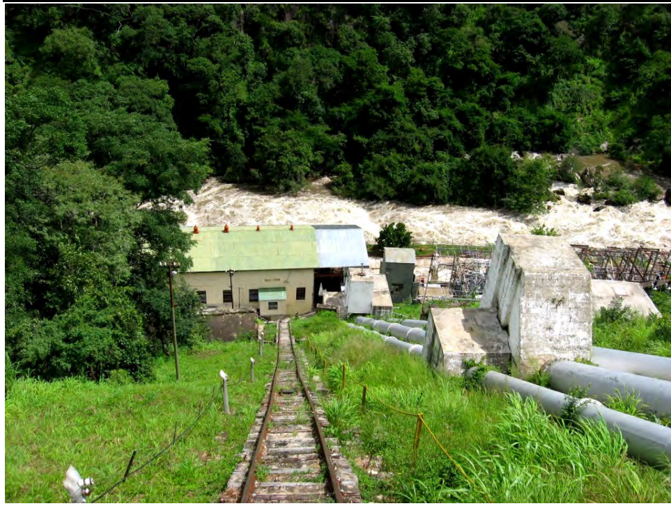
Figure 4.22 Existing Mulungushi Powerhouse: External view (from funicular rail)
